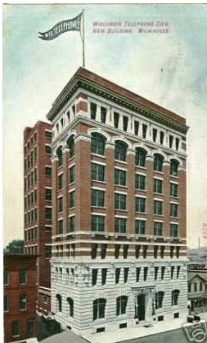
Figura 3.38: Wisconsin Telephone Co. , Milwaukee, Alexander Eschweiler 80 , 1905-1907.
