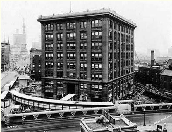
1930 Indiana Bell Telephone Building on the move
