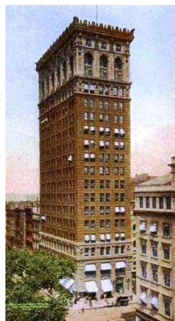
Figura 3.35: Chambers Building , 1889-1890, Cass Gilbert.
