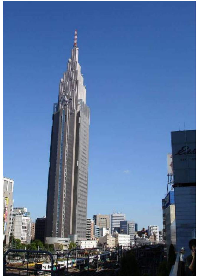
Figura 6.19: NTT DoCoMo Yoyogi Tower, Tokyo, 1997-2000, NTT Power and Building Facilities. Fotografía: Lye Gunnstein.
