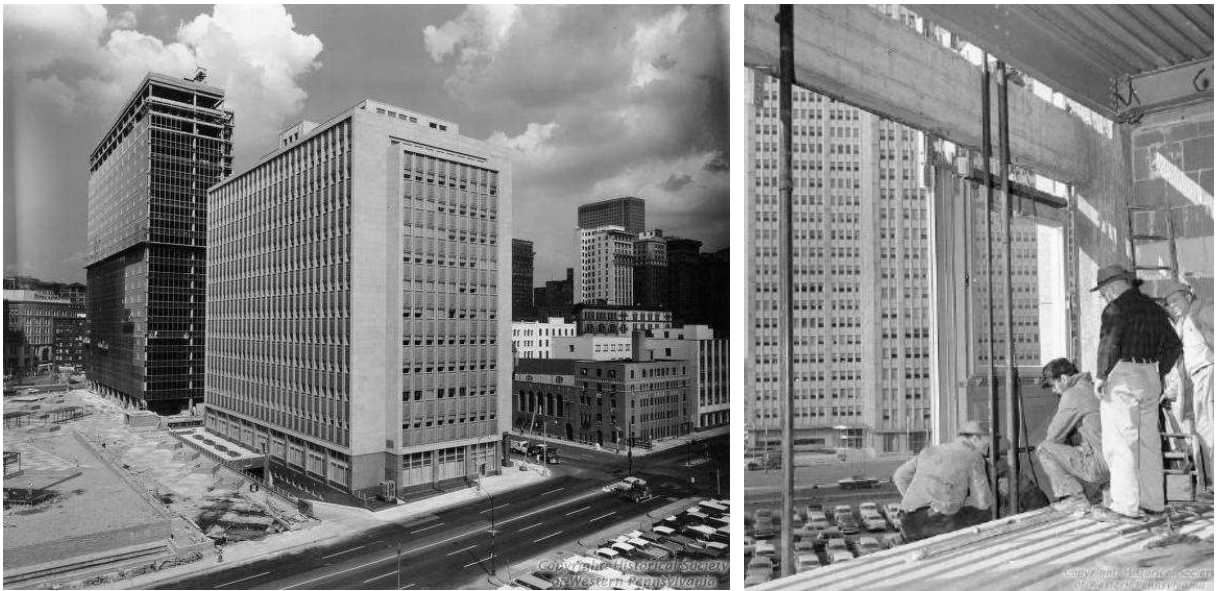
Figura 5.37: Bell Telephone Company Building, Pittsburgh (Pennsylvania), 1956-1957, Press C. Dowler y William C. Dowler.
