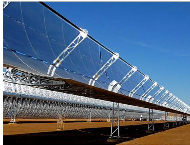
Fig. A3. Concentration scheme through a parabolic cylinder mirror. Source: [78].
