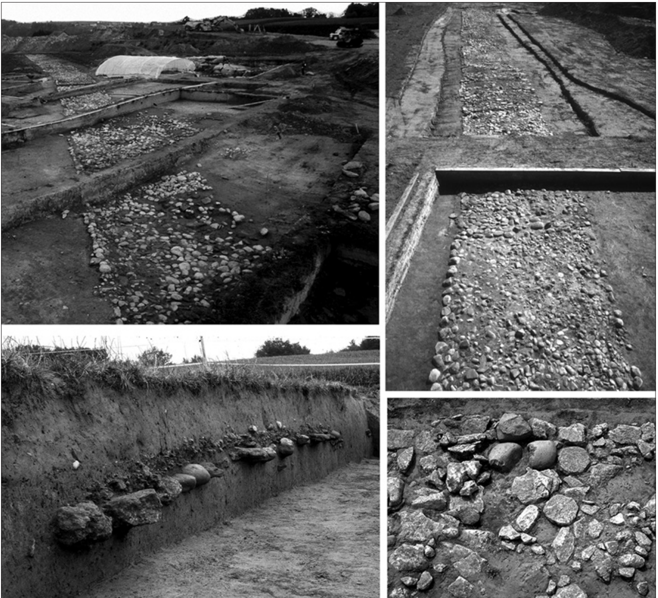
FIGURE 3. THE ROAD. CLOCKWISE FROM UPPER LEFT. A: GENERAL VIEW FROM THE WEST REVEALING ITS SLIGHT CHANGE OF DIRECTION AFTER THE FORD; B: VIEW FROM THE WEST OF THE ROAD'S EASTERN SEGMENT; C: DETAIL OF CYLINDRICAL QUERN ROUGHOUTS FROM THE QUARRY SERVING TO REPAIR THE ROAD; D: CROSS-SECTION OF THE ROAD REVEALING ITS STONE FOUNDATION AND CONVEX GRAVEL COVER (FROM ANDERSON ET ALII 2003)
