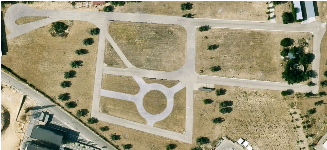
Fig. 6. Private driving circuit at CAR.
