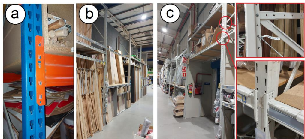
Figure 5. (a) Beam–end connection to perforated profile column in steel storage racks, (b) load-bearing structure made of steel racking, and (c) steel racking from perforated profiles.
