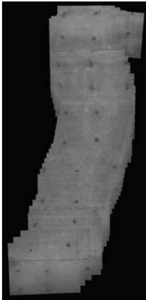
FIGURE 13. Mosaic image of the upstream dam wall
